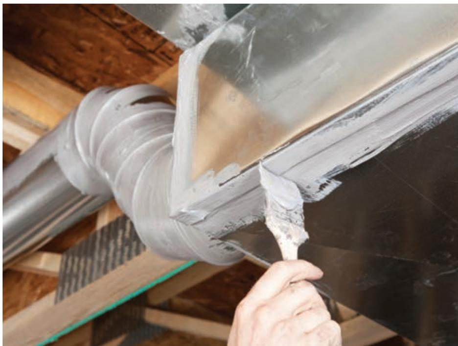
**Need to seal your ducts? Don't reach for the duct tape. Use a mastic sealant or metal tape.**
