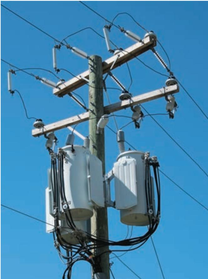
**Transformers lower the high voltage of electricity as it makes its way through the system, making it safer for distribution to your home.**
