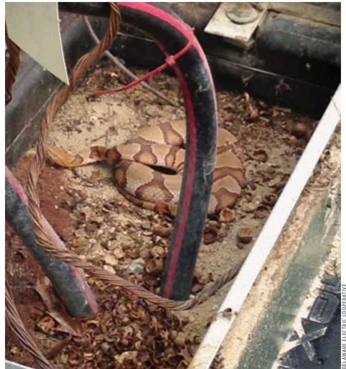
Snakes (like this copperhead) and rats turn a neighborhood's green, pad-mount transformers into cozy dens. The transformers switch electricity from 12,500 to 240 volts. When animals gnaw on wires inside the transformer, they get hurt and cut power.
