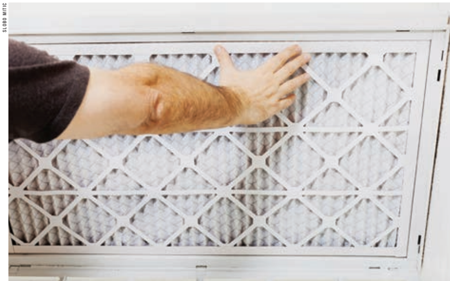
Regular maintenance for your air conditioner, including checking for a clean filter, will help it run more efficiently.
