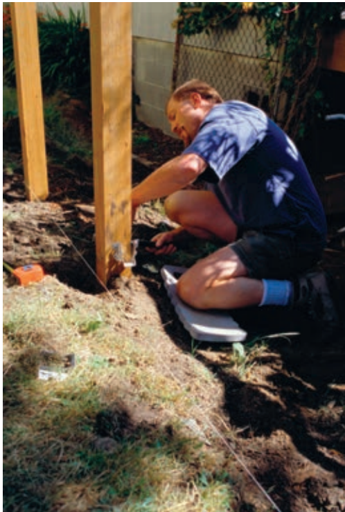
Adding a fence or repairing a deck? Be sure to call 811 first to make sure there are no underground utilities that might get in the way.
